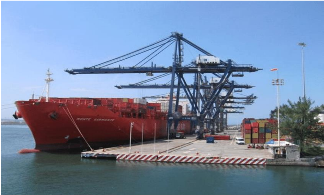
Fig. 1: Harbor facilities made by structural steel [4]
